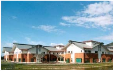
Port Talbot Hospital, Neath
